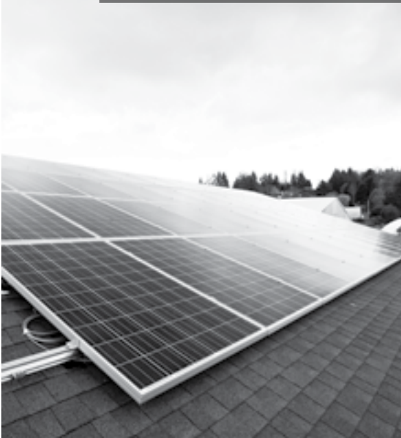
Solar panels on the roof of the sprouting facility. Credit: Pamela Powell.
