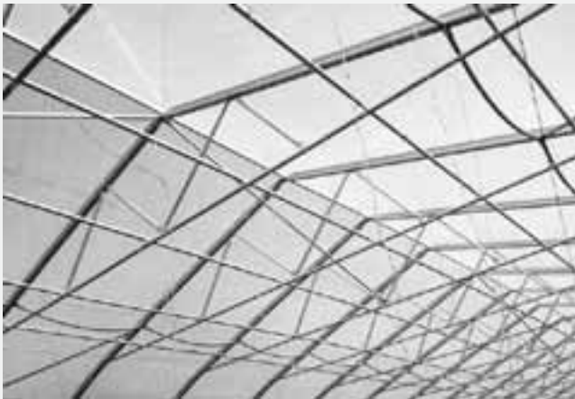
From top to bottom: 1. Additional bracing on the coldframe sides help distribute energy from wind gusts to the second and third arches. Additional corner bracing prevents distortion of corners, helping to maintain 90 degree angles. 2. Diagonal bracing extending from above the doorway up to the peak of the second arc helps distribute energy from wind gusts across the structure. 3. The diagonal bracing starting at the top of doorways continues throughout the structure, adding strength and helping to distribute energy across the entire structure. Credit: Chris Bodnar
