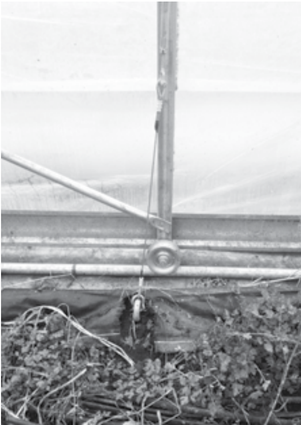
Left: detail of wheel and rail that makes this coldframe move. Right: anchoring system. Credit: Chris Bodnar
