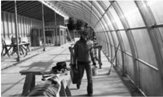
The Common Greenhouse under construction Photo Credit: Lin Steedman
